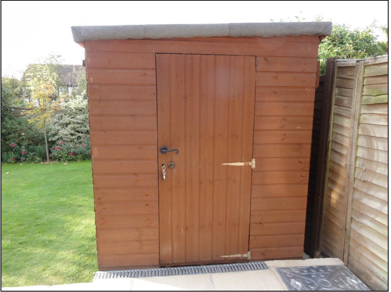
The door and the fixed roof fitted and felt fitted.
