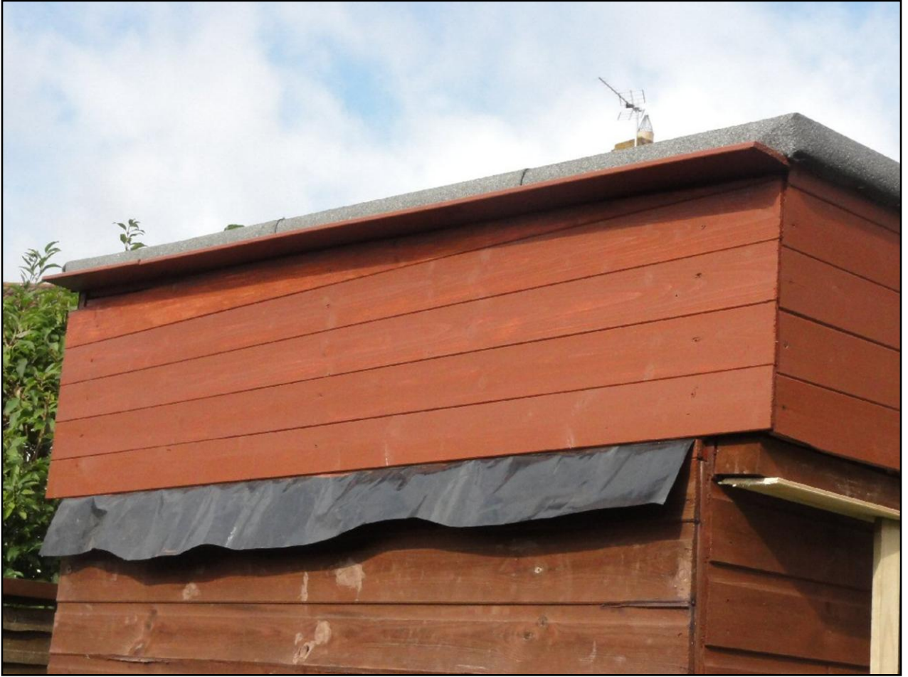
The low viewing / ventilation flap fitted into position with the rain seal sheet.
