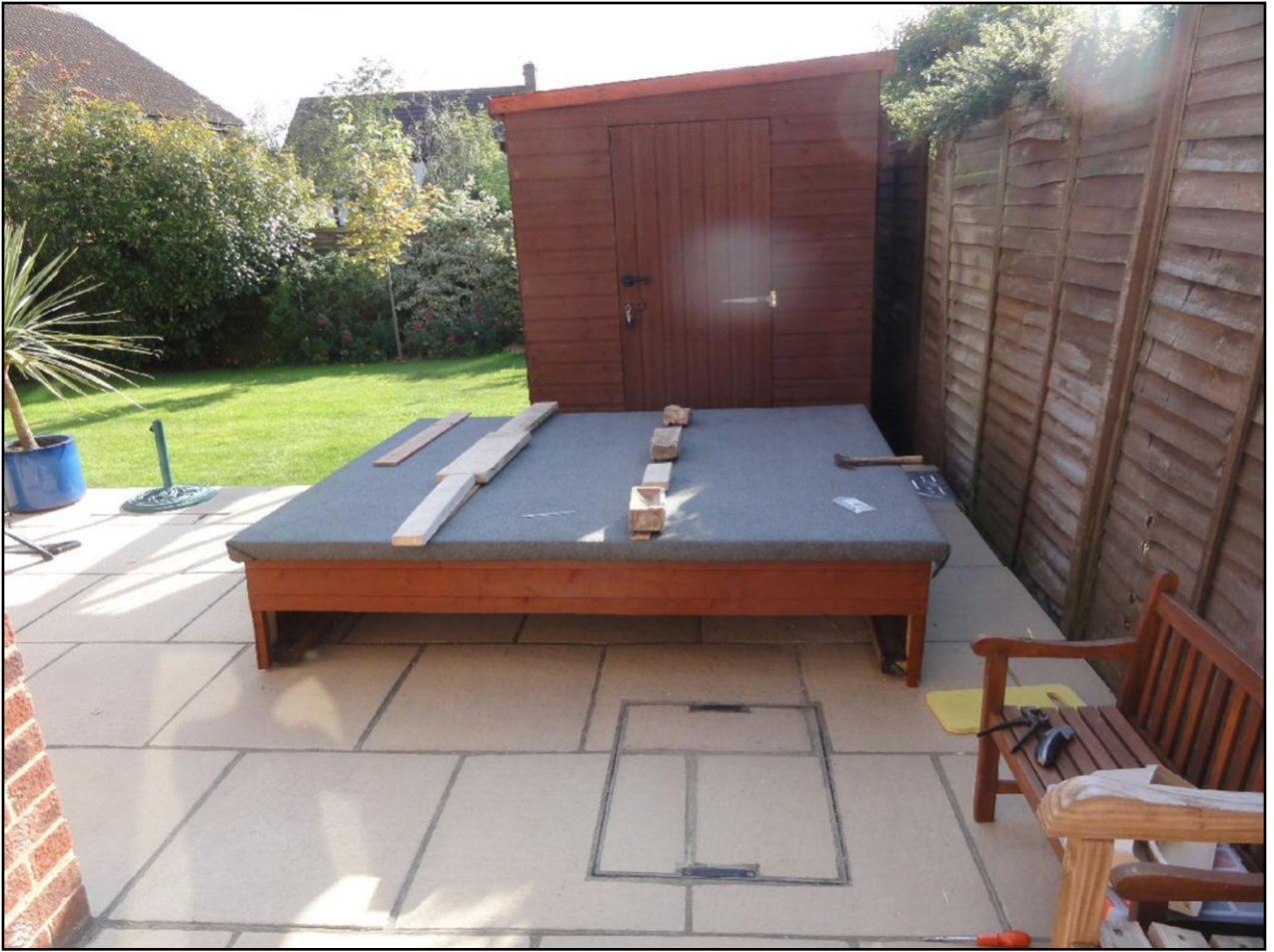
Fitting the sliding roof felt.
