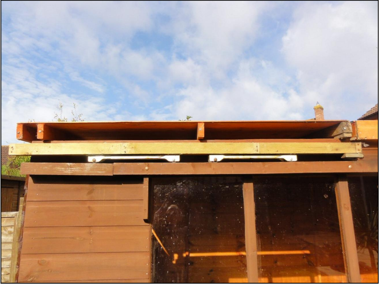
Checking the original roof half and the sliding roof support trolleys.
