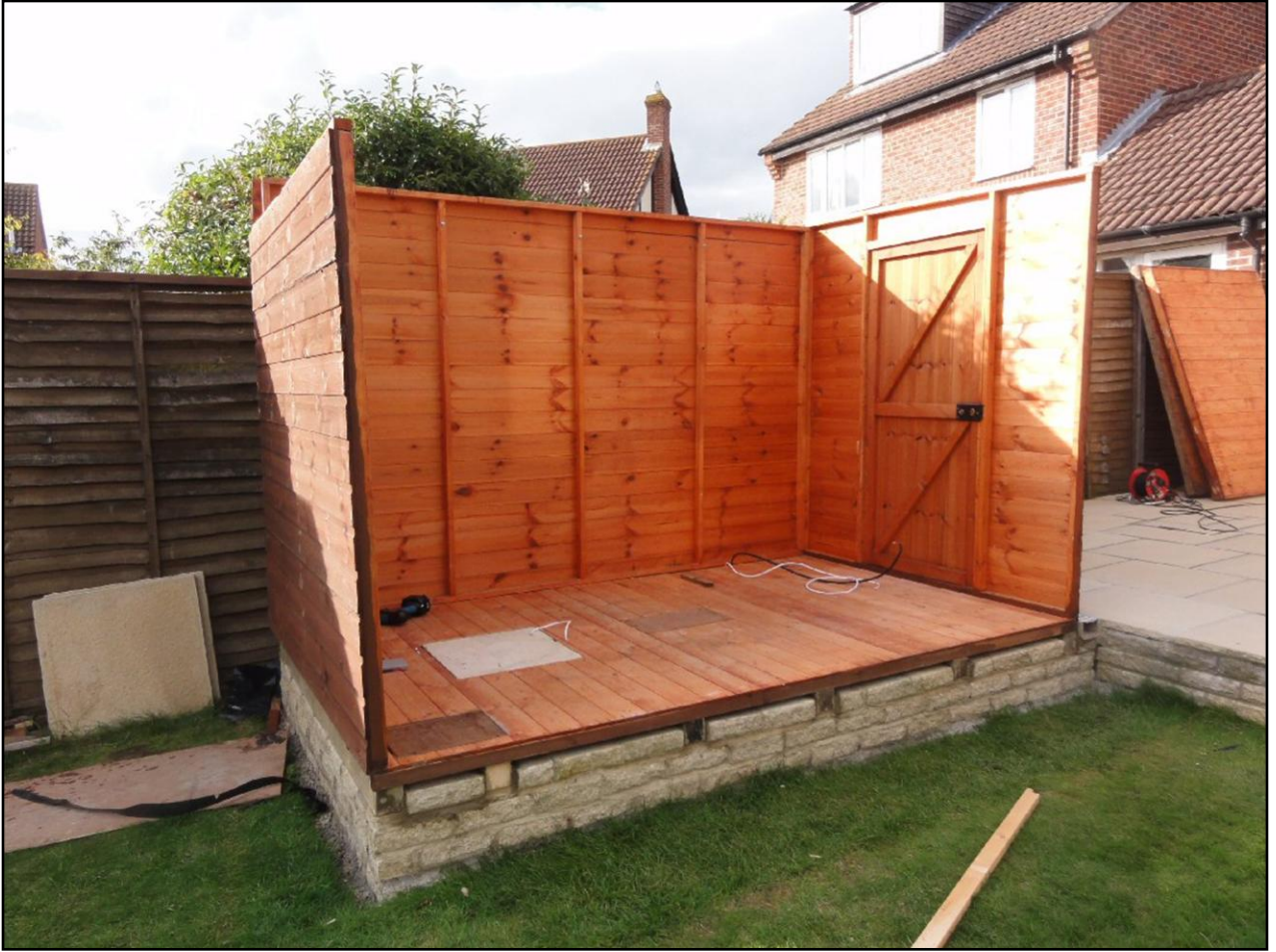
The walls were then fitted and secured to the floor.
