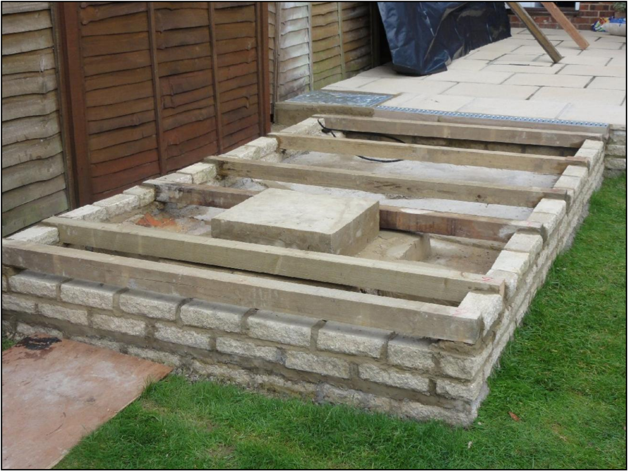
The foundations and floor supports are in place and ready for fitting the floor.
