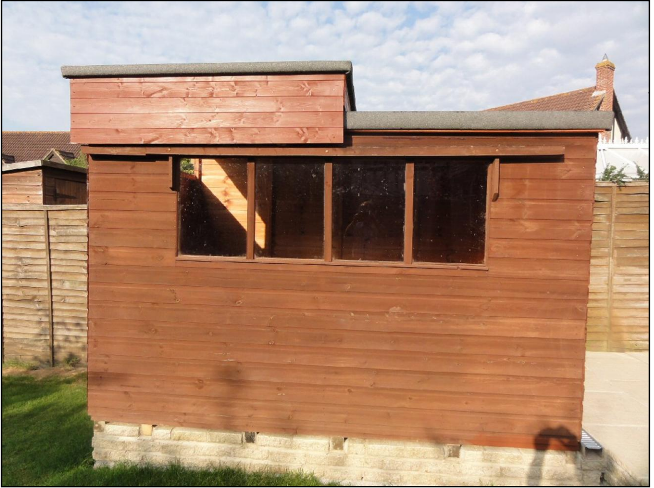
The sliding roof lifted on to the runners and slid forward to butt against the stop and sealing bar.
