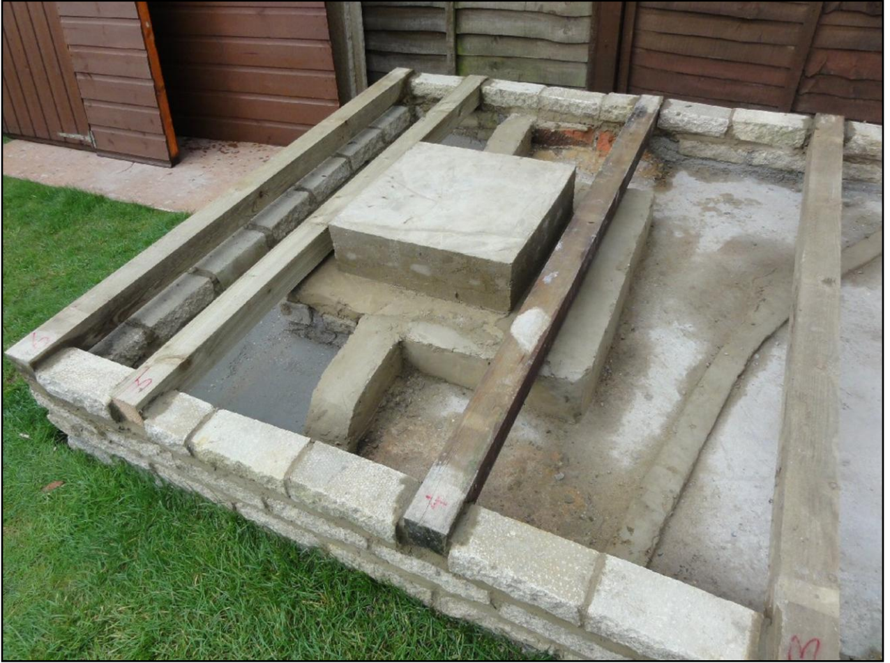
The floor support beams were fitted and secured in place.
