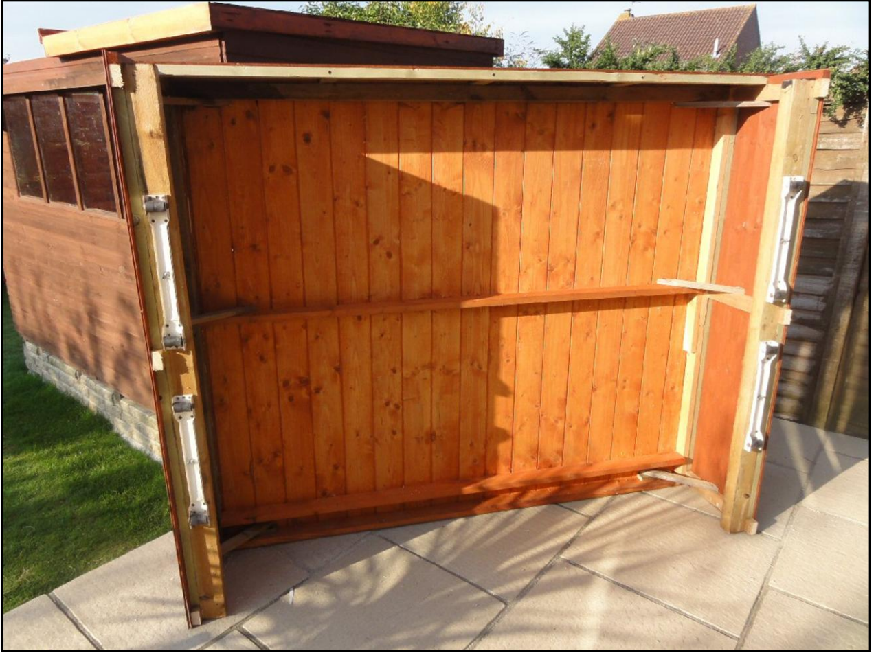
Assembling the new sliding roof with its side support walls and trolleys.
