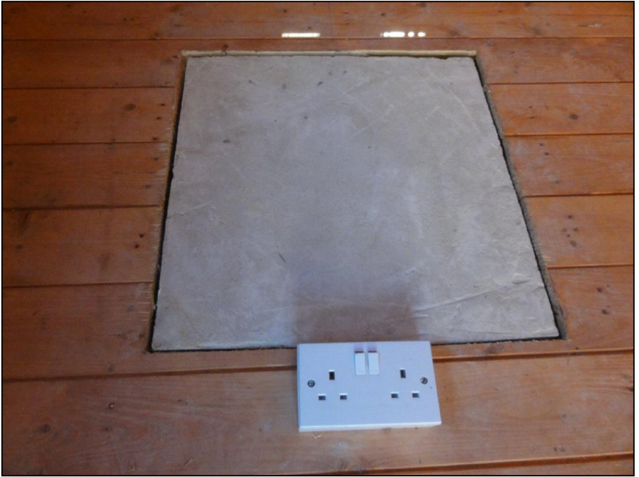
The floor mounted mains electrical sockets fitted.
