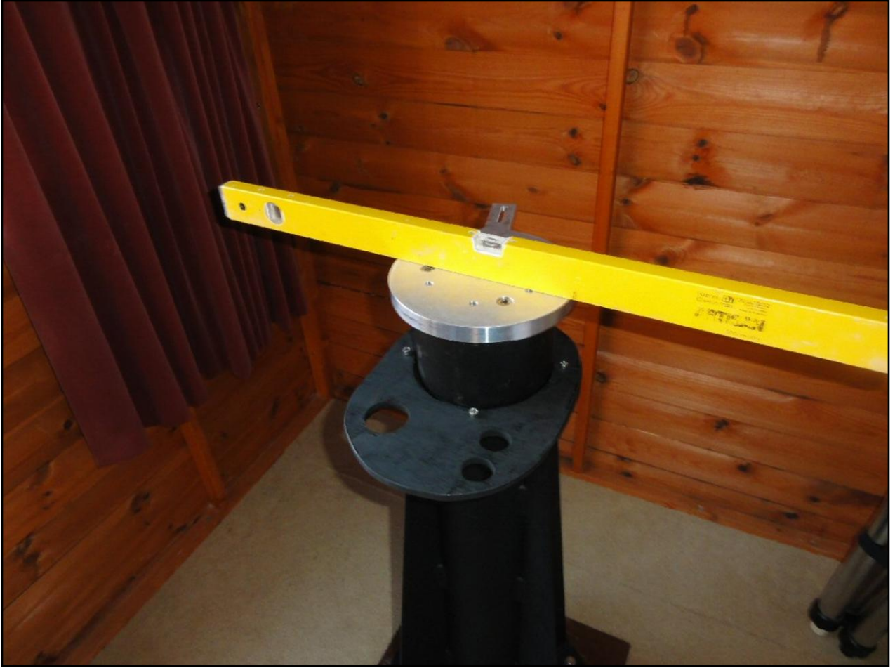
Checking the level of the pier assembly.
