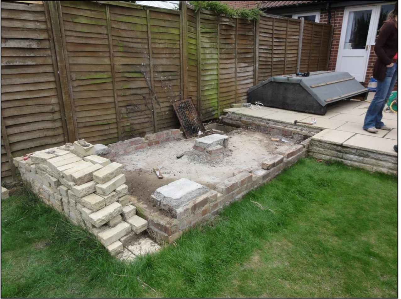
The rear (south) foundation wall was to be moved 600mm down the garden.
