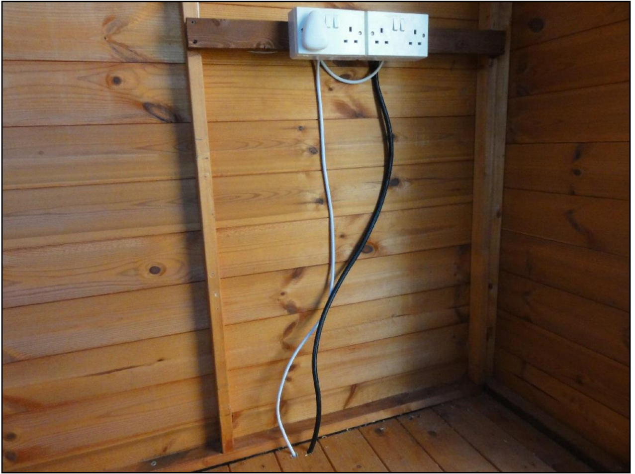
The wall mounted mains electrical sockets fitted.
